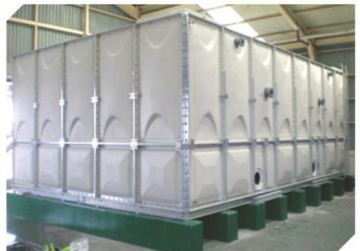
Completion of Installation Assembly panels with steel reinforcement members on site
